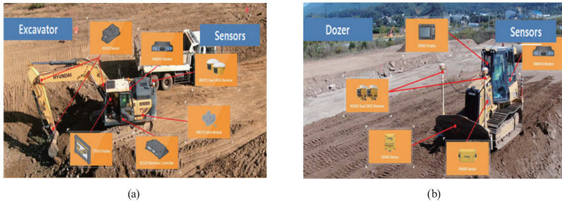
Fig. 15. (Color online) Construction equipment and sensors. (a) Excavator. (b) Dozer.
