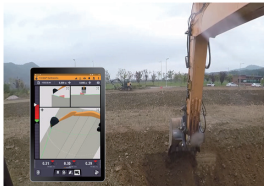
Fig. 16. (Color online) Work screen for automated construction.
